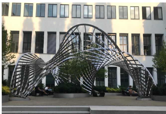
Fig. 1.1. ‘Asymptotic Gridshell’ forms the INSIDE\OUT pavilion. (Picture: Hui Wang)
